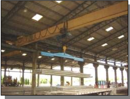
Over Head Crane
